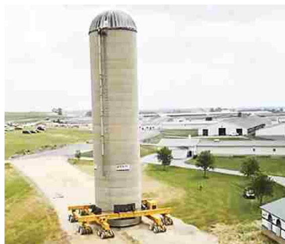
Figure 45: Moving of a silo at Kreider Farms in Manheim, PA to create an observation tower
